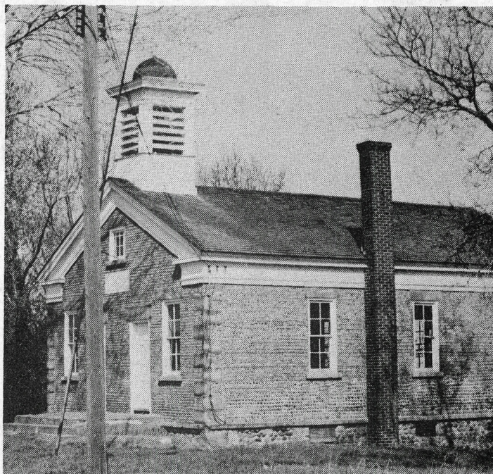
DISTRICT NO. 5 -- Cobblestone school house in Childs is from late period, built around 1849.
